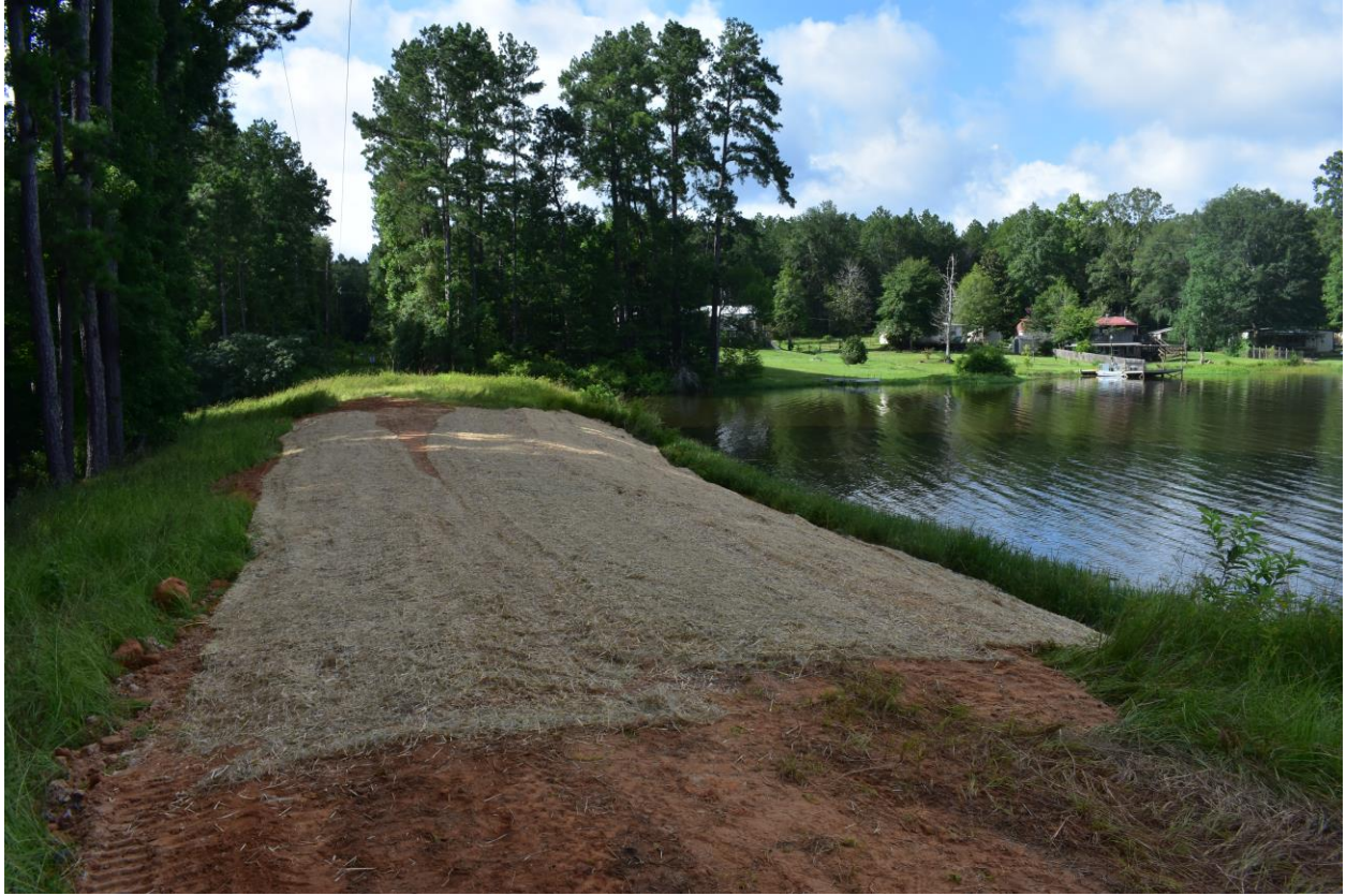
Figure 19 - Low area close to the spillway. After the erosion control mat
