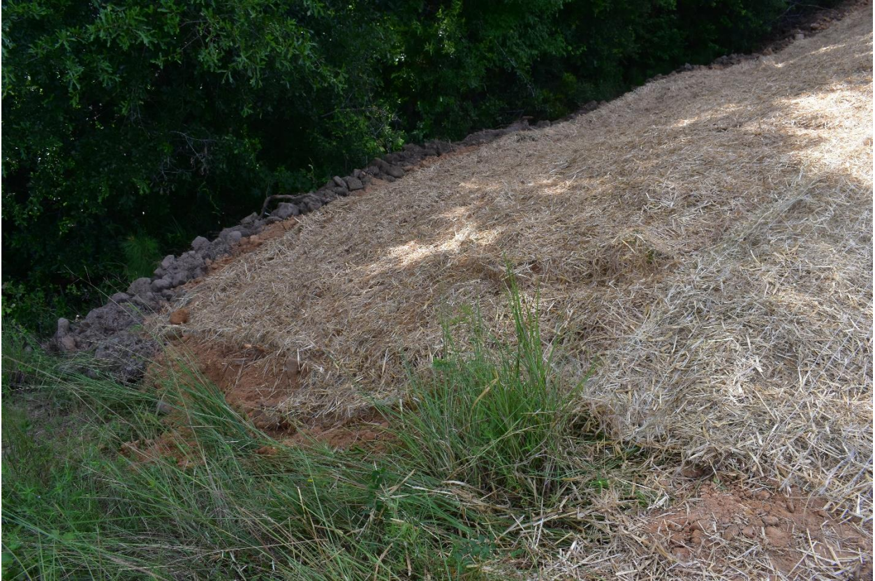
Figure 24 - Back side of the dam around the low flow pipe. After the erosion control mat
