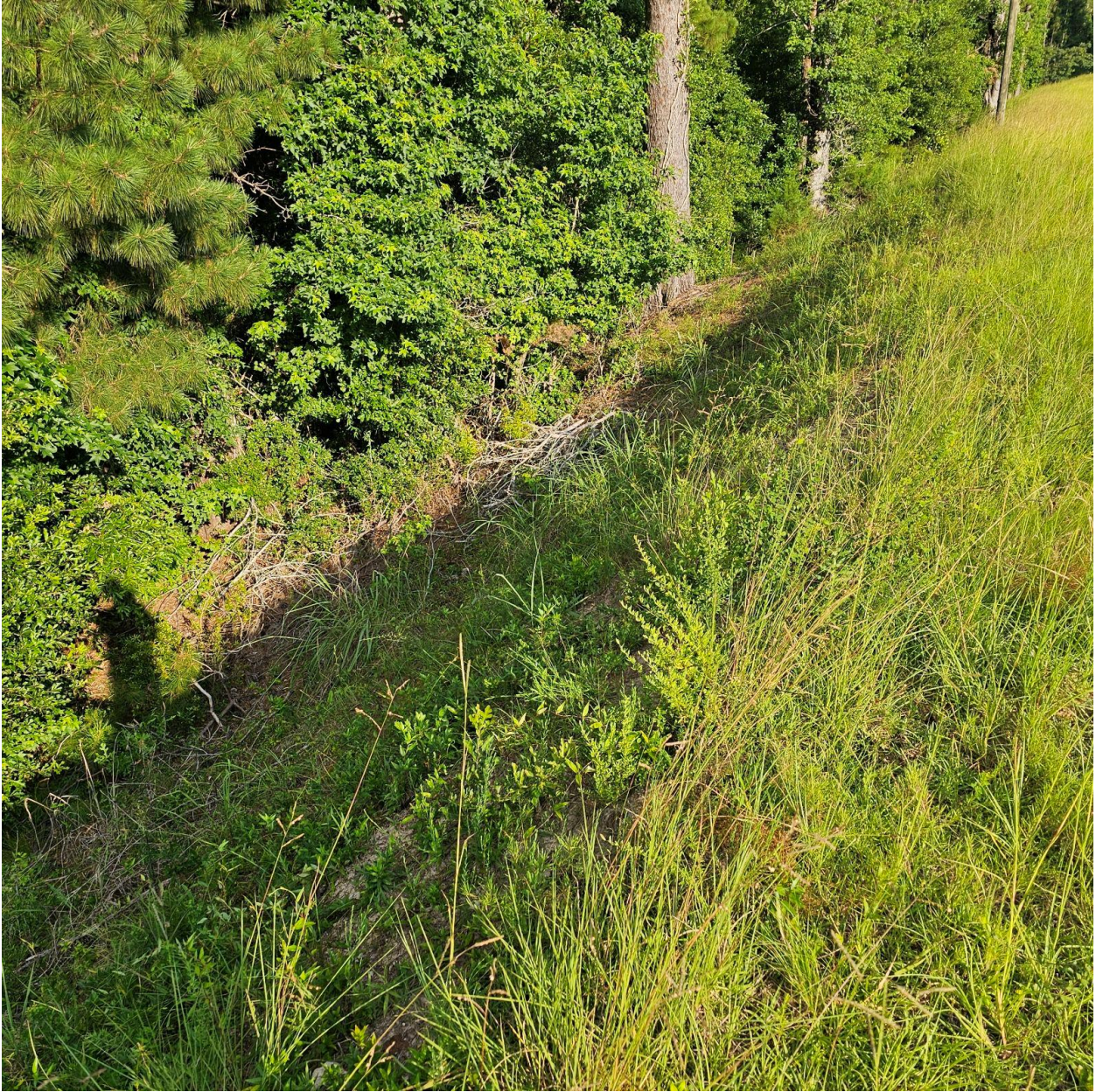
Figure 1 - Back of the dam around low flow pipe facing South. Before work was done
