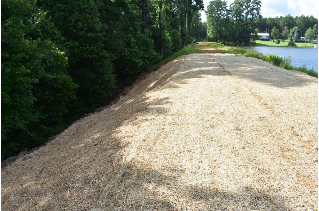
Figure 23 - Back side of the dam around the low flow pipe. After the erosion control mat
