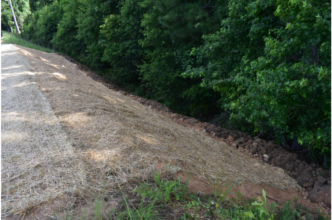
Figure 22 - Back side of the dam around the low flow pipe. After the erosion control mat
