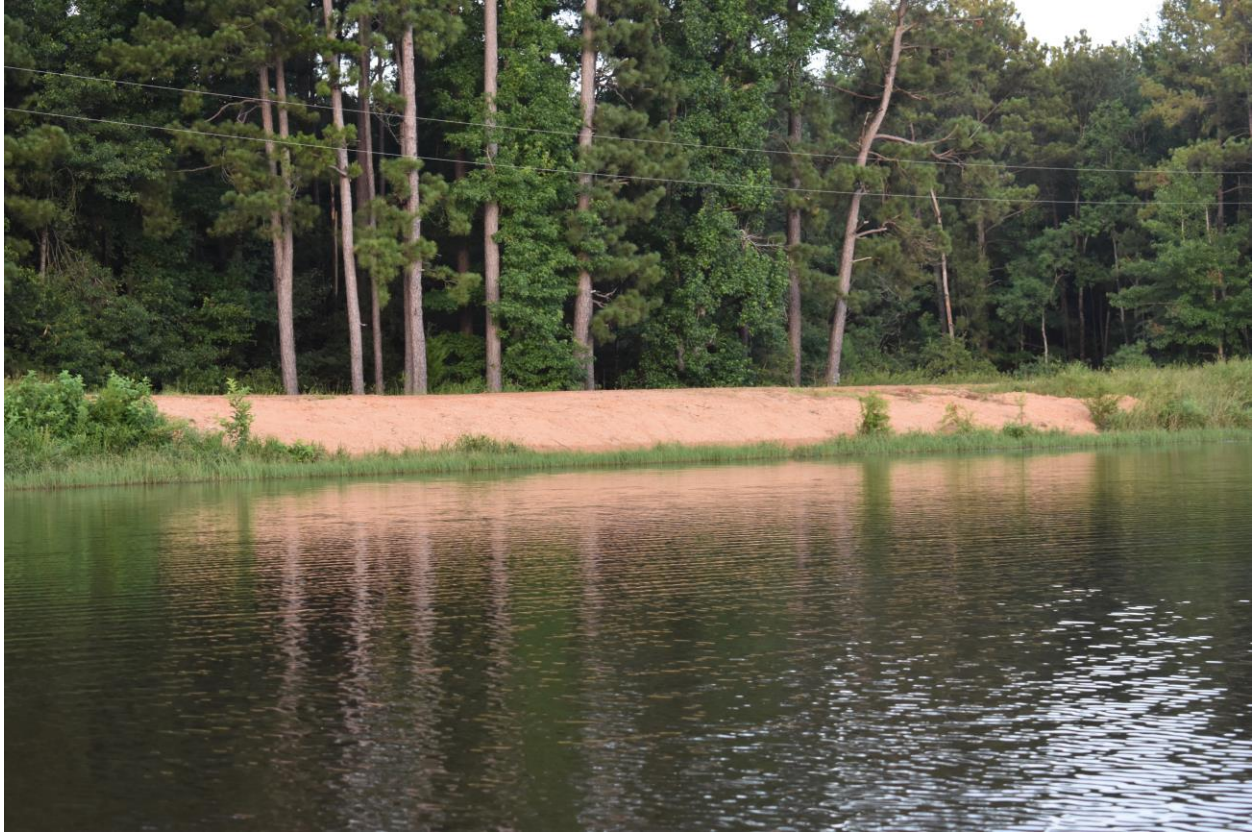
Figure 14 - Low area close to the spillway Before erosion control mat
