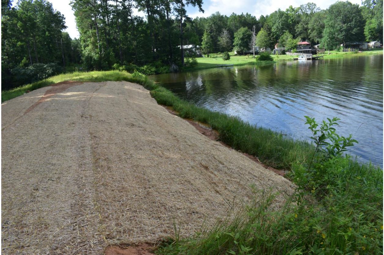
Figure 20 - Low area close to the spillway. After the erosion control mat
