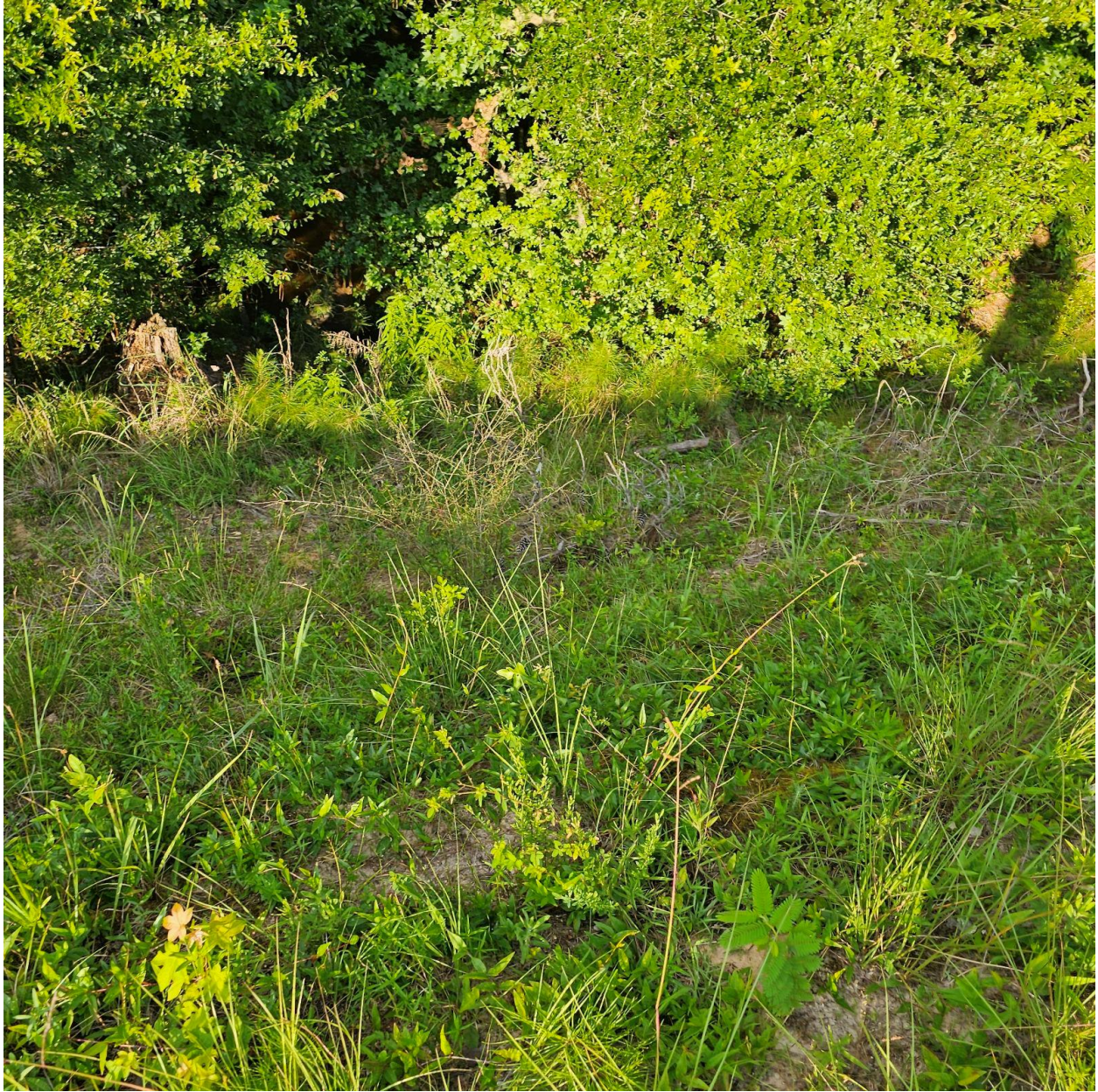
Figure 2 - Back of the dam around low flow pipe. Before work was done
