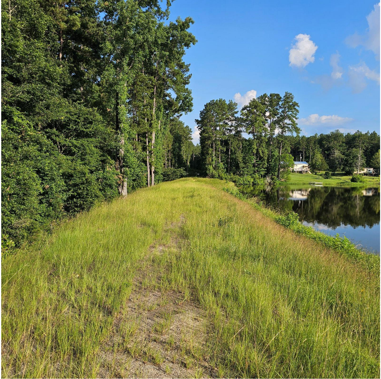
Figure 4 - Top of the dam around low flow pipe facing South. Before work was done
