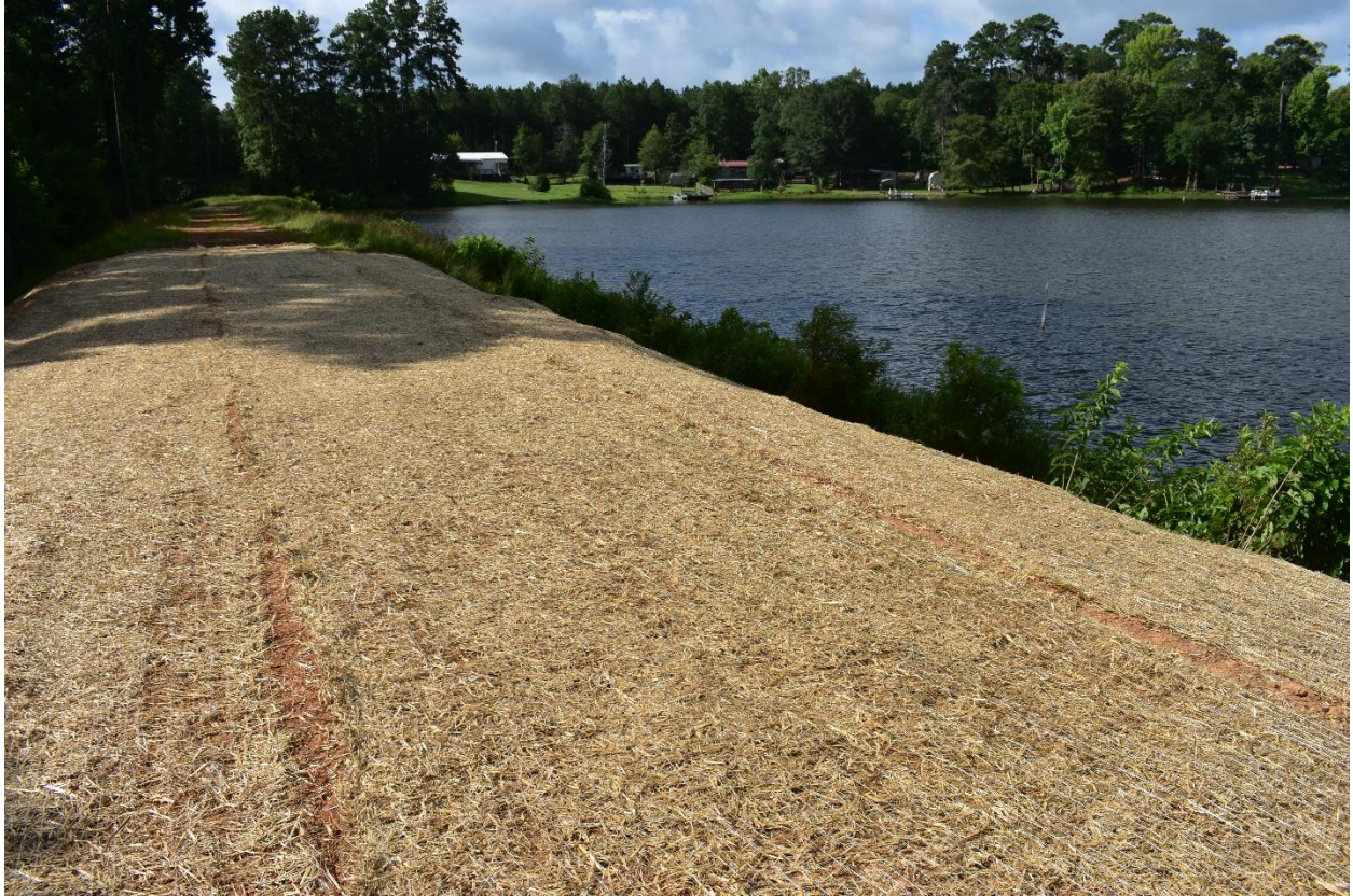
Figure 24 – Top side of the dam around the low flow pipe. After the erosion control mat
