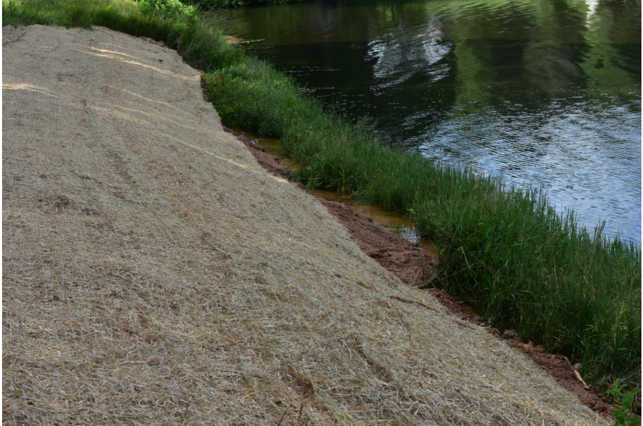
Figure 21 - Low area close to the spillway. After the erosion control mat
