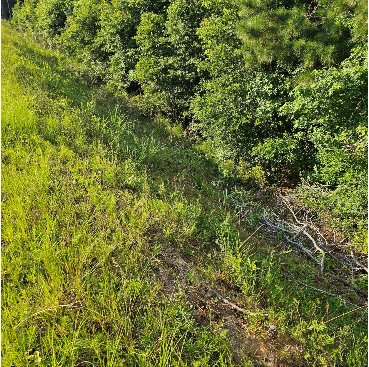
Figure 3 - Back of the dam around low flow pipe facing North. Before work was done
